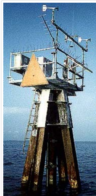
Coastal-Marine Automated Network (C-MAN) Station.
